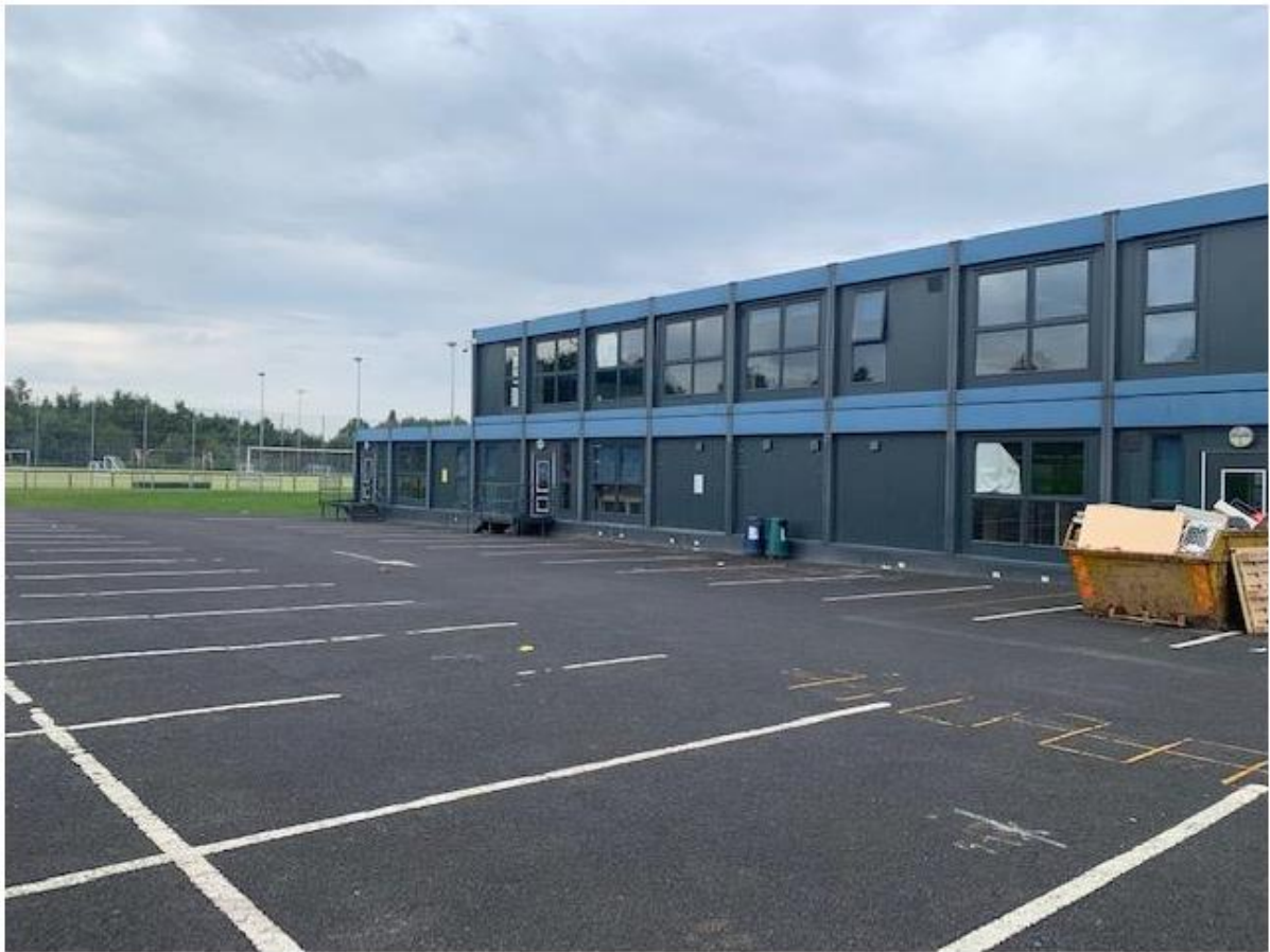
Photo 4: Existing temporary modular buildings (to be removed/demolished)
