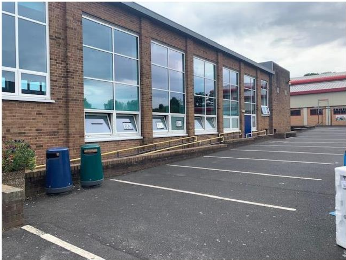
Photo 2: Existing school elevations
